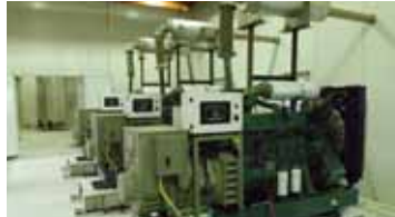
Utilities - HVAC & pump rooms
