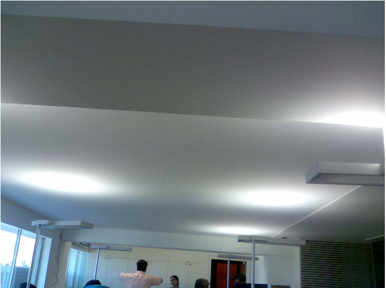
'Stretch SLS as an energy saving light reflector – Era Architects office, Mumbai, India
