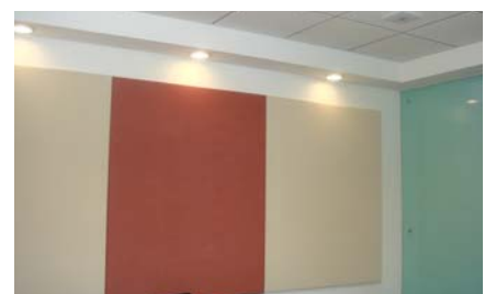
ACT KLH installed modularly in two-tone colours
