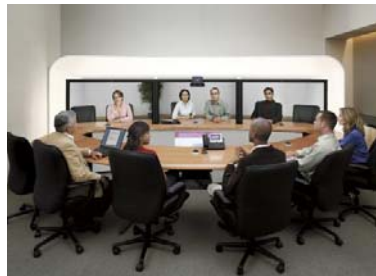
Curved tables and screens in a matching curved configuration make for comfortable sightlines. Note the pop-up touchscreens for meeting controls and/or multitasking
